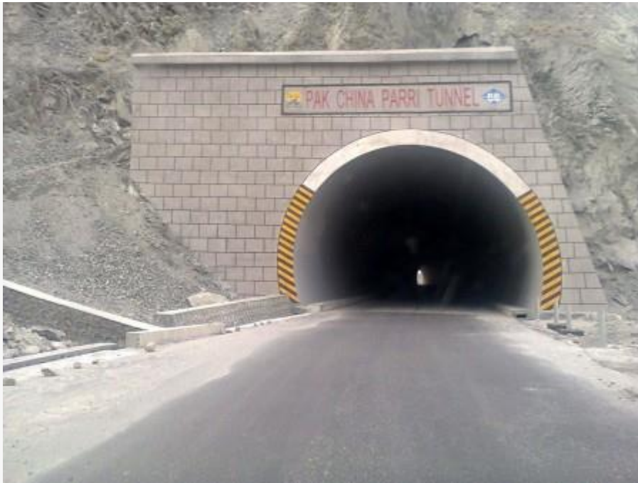
A recently inaugurated tunnel located between
